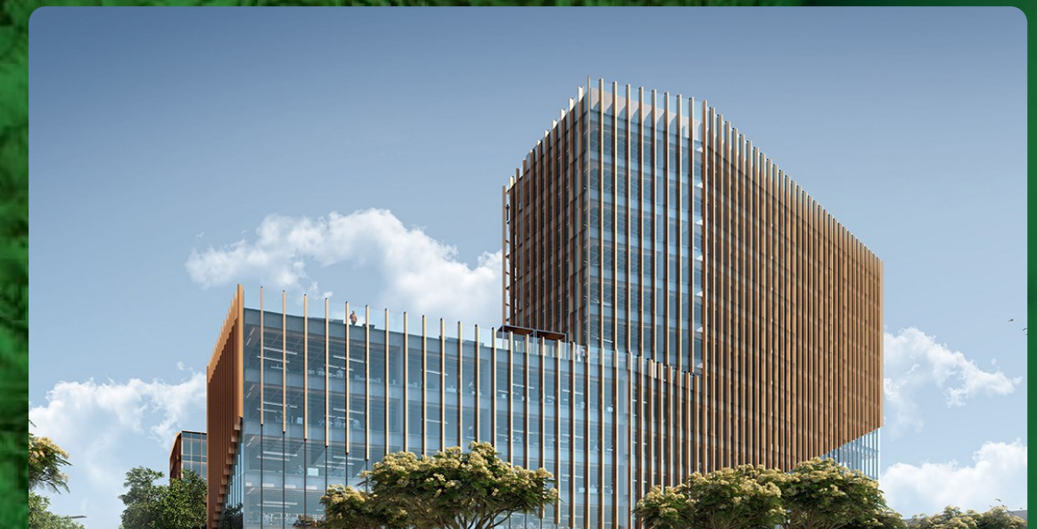
EXEO OFFICE CAMPUS - LISBON
