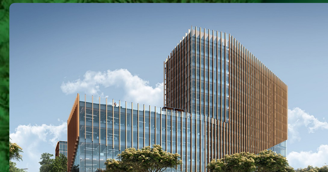
EXEO OFFICE CAMPUS - LISBON
